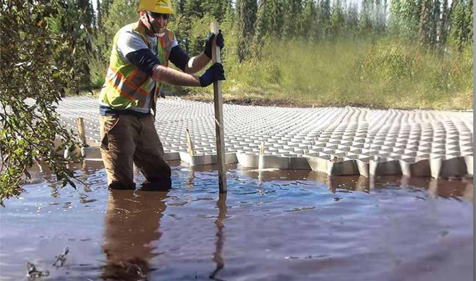
Access road design for MEG Energy using NPA Geocells eliminated the need for muskeg (peat) removal, dewatering, disposal, and soil replacement, and reduced the need for imported aggregates.
