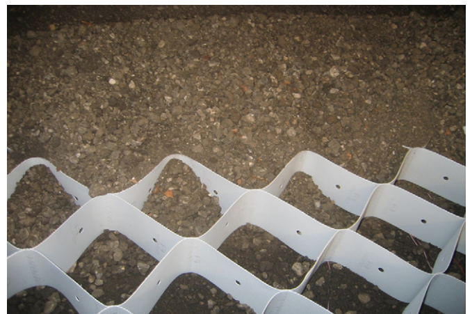
Fig. 1. Geocell infilled with RAP.
