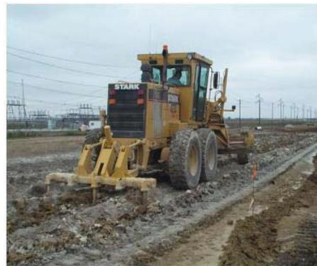
Fig. 2 Mixing of the lime by a tractor
