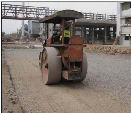
Fig. 5 Compaction by a vibro roller
