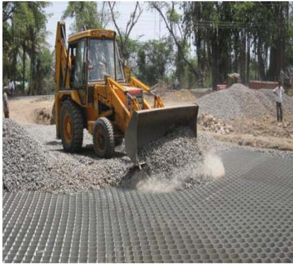
Fig. 4 Filling the geocell pockets
