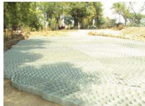
Fig. 3 Geocell layer spread over the road section
